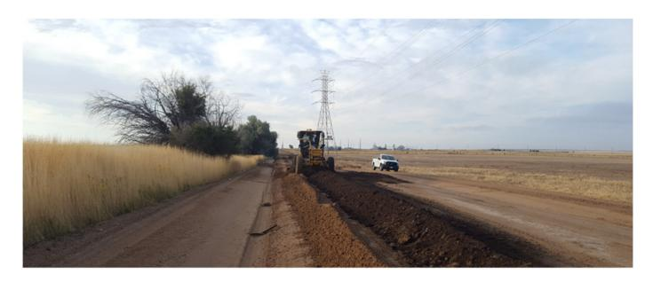
When necessary, re-establish proper road elevation for drainage and cross-section crown. Build hard stable sub-layer capable of supporting traffic loads and reduce susceptibility to adverse weather affects and wash-out erosion.
